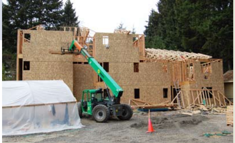
White Caps Apartments under construction.
